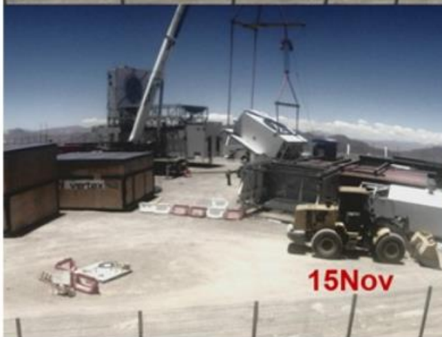
Installation of the FYST yoke arms on 10 Nov (top) and 15 Nov (bottom). Notice the yoke traverse was rotated 180° between the two dates. Nov 2025
