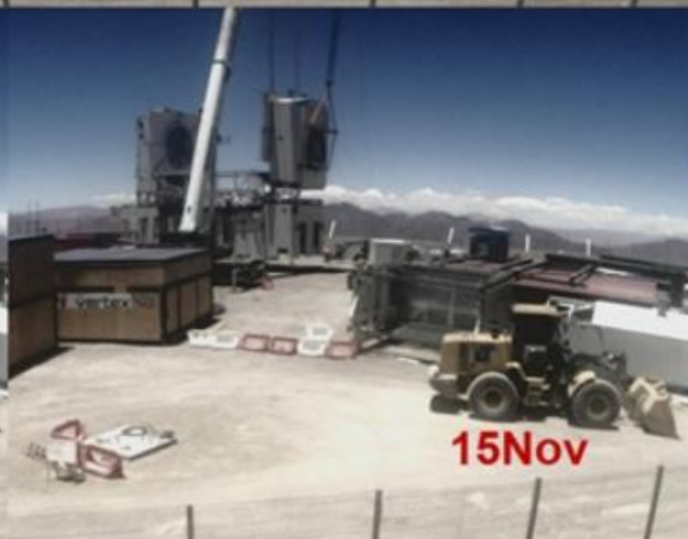
Installation of the FYST yoke arms on 10 Nov (top) and 15 Nov (bottom). Notice the yoke traverse was rotated 180° between the two dates. Nov 2025
