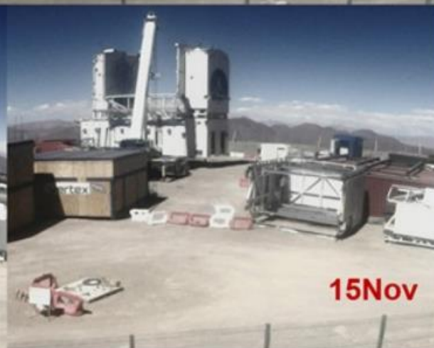
Installation of the FYST yoke arms on 10 Nov (top) and 15 Nov (bottom). Notice the yoke traverse was rotated 180° between the two dates. Nov 2025
