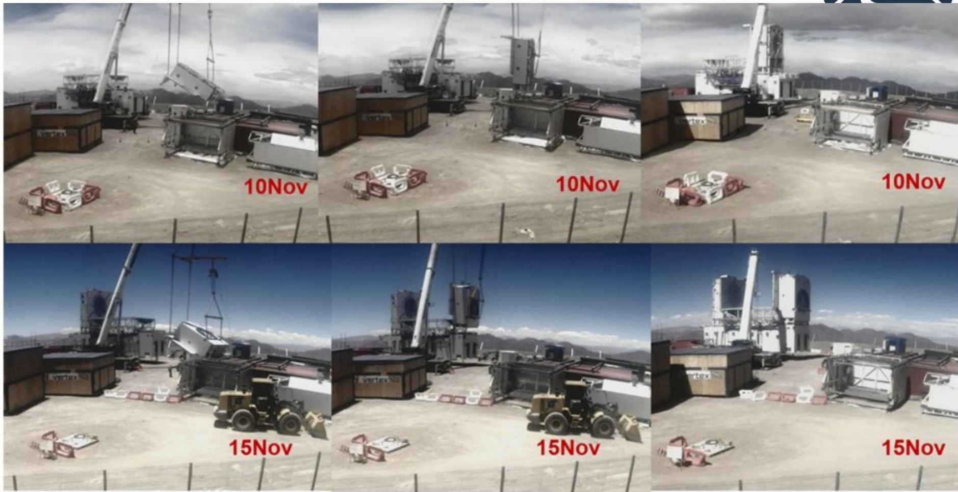
Installation of the FYST yoke arms on 10 Nov (top) and 15 Nov (bottom). Notice the yoke traverse was rotated 180° between the two dates. Nov 2025
